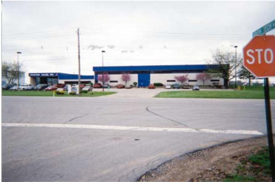
SR-741 at South Tech Blvd looking east
