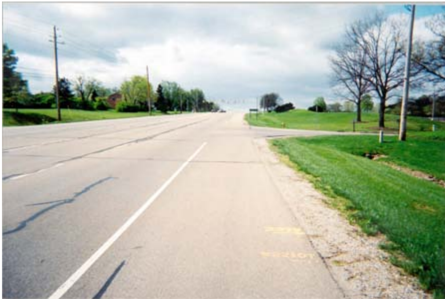
SR-741 north of Miami Village Dr looking south
