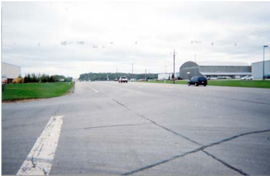
SR-741 at South Tech Blvd looking north
