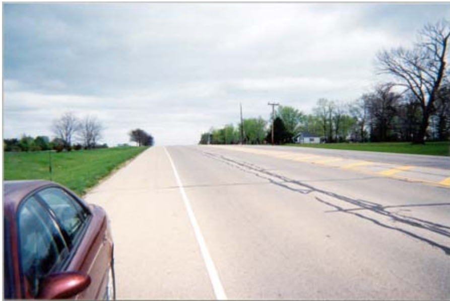
SR-741 south of Wadruhe Park looking north
