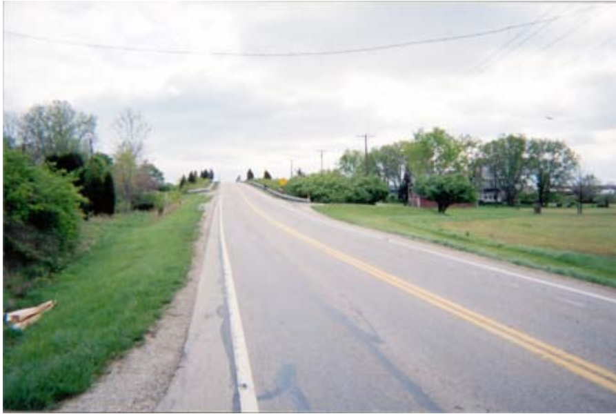
Miamisburg-Springboro Pike east of Byers Rd looking east
