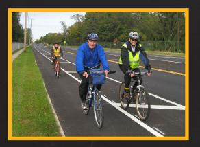
A buffered bike lane is a lane with additional space—a buffer—between bicycles and cars. Bicyclists ride in the bike lane and motorists drive to the left of the buffer.
