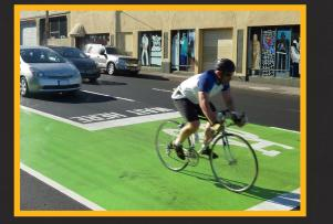
A bike box is a green marked pavement area at a road intersection with a white bicycle symbol inside it.
