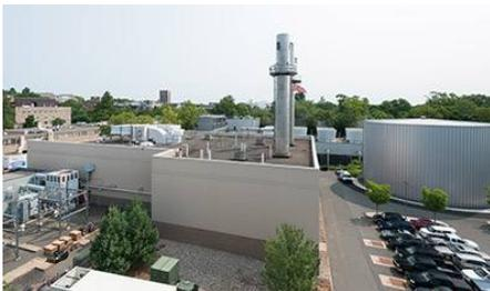
The heart of the Princeton microgrid is the cogeneration plant (center), which was constructed in 1996. The plant produces electricity as well as steam used for heat, hot water and sterilization. The plant also runs the industrial "chillers" that cool the 2.6 million gallons of water used to cool campus buildings and research instruments such as
