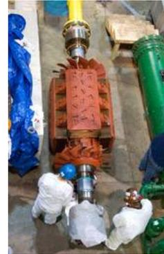
Two years after Hurricane Sandy, Princeton University's "microgrid" power generation and distribution network is a national example of how to keep power running for residents, emergency workers and crucial facilities when disaster strikes. Pictured is the microgrid's main generator, which is powered by a natural-gas turbine.
