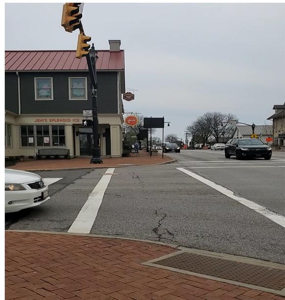
Image 12: The tactile panels are not ADA-compliant.
