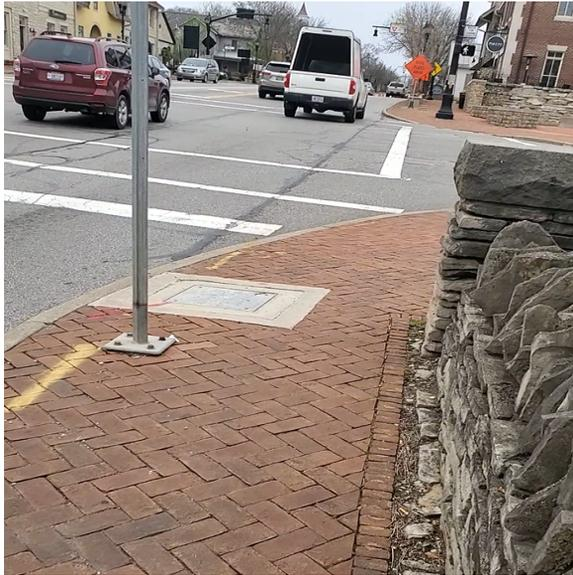
Image 9: The intersection at High Street and Bridge Street includes well-marked crosswalks. Tactile panels are not ADA-compliant. A Dublin walk audit participant suggested implementing a scramble light for this intersection.
