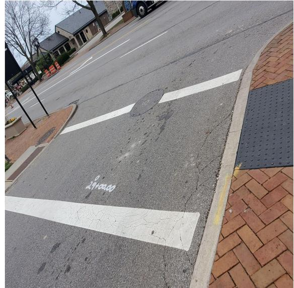
Image 2: Tactile panels are in the direction of travel.
