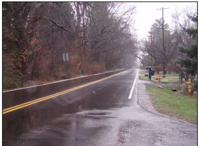
Shoulder widening would necessitate relocation of signs and mailboxes in some locations
