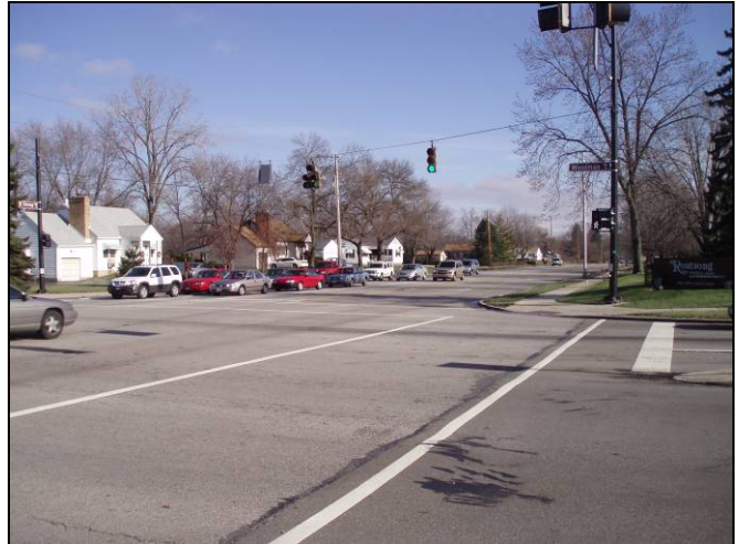
Lower-visibility crosswalk markings characterize the Stroop Road/Woodman Drive intersection
