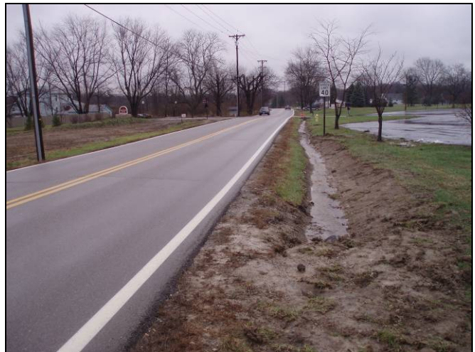
The addition of bike lanes and sidewalks/pedestrian paths would require culverts, bioswales and/or other treatments to address drainage issues
